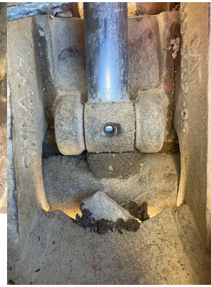
Image Comment(s): Coupler cylinder pin grease nipple broken. Grease nipple replaced.
