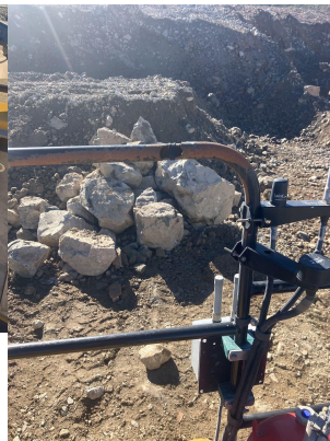
Image Comment(s): Left rear handrail broken.
