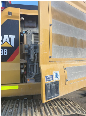
Image Comment(s): Left cooler door cracked.
