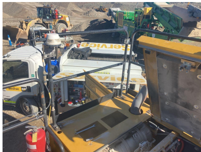
Image Comment(s): Right rear handrail loose. Mounting bolts tightened.
